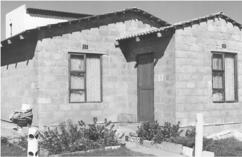
Figure 3.13: Lizzie Mgedezi's house in Hazeldene, next to VM, completed in 2002.
