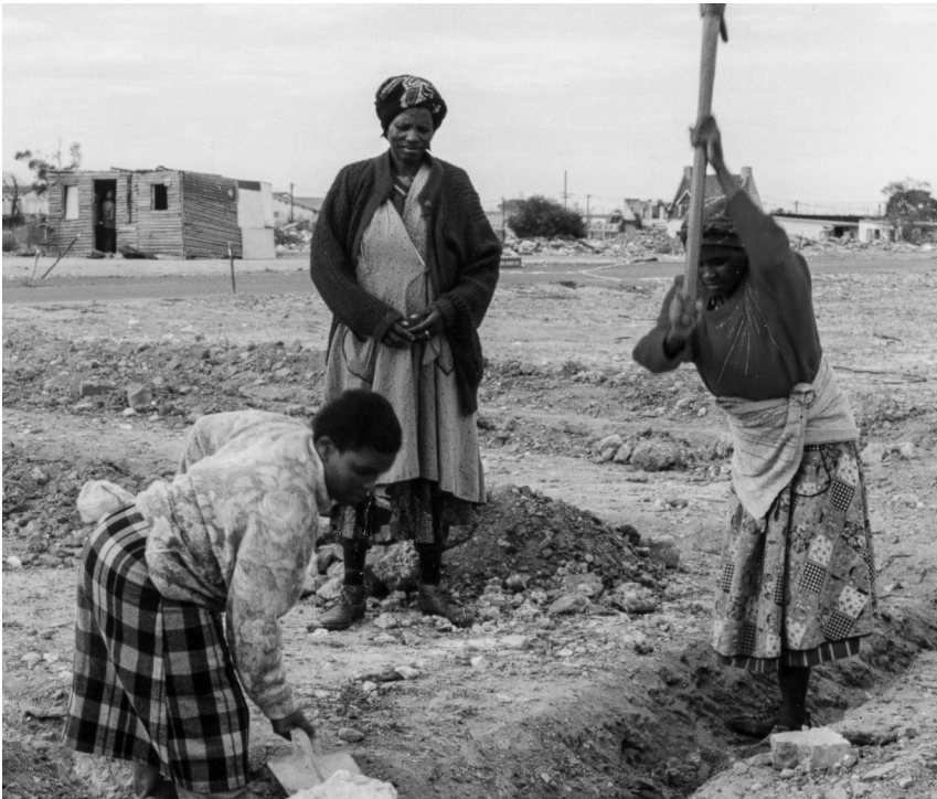
Figure 3.8: Women digging the first foundations.
