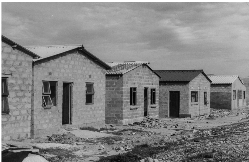
Figure 3.15: The VM houses are almost ready.
