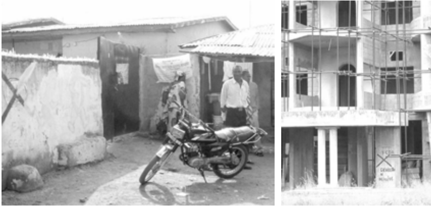
Figure 4.1: Planned demolition—crosses on a crèche in Lugbe, one of Abuja's 'slums', and on a multi-storey building in central Abuja
