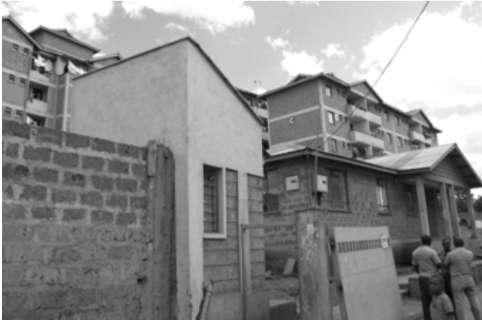
Figure 6.8: The Langata decanting site
