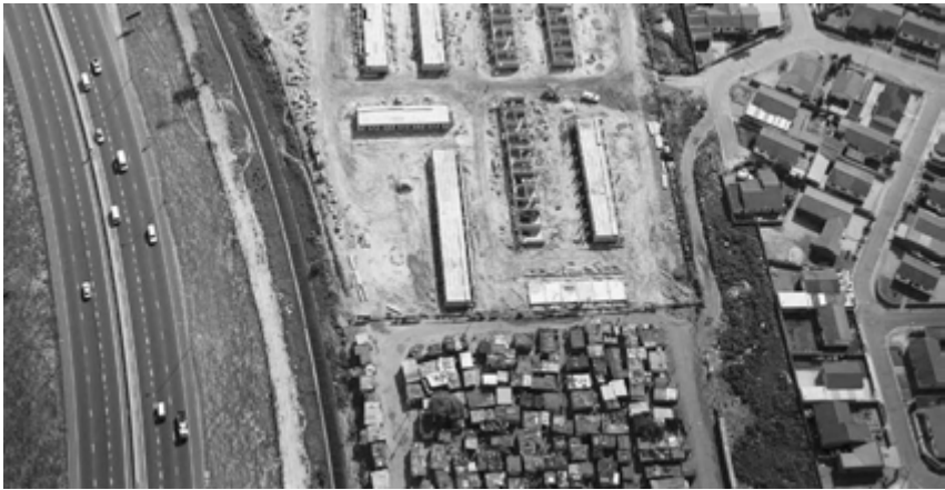
Figure 6.3: Phase One of the N2 Gateway Project under construction in 2005
