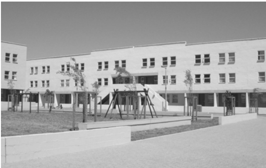
Figure 6.4: Rental housing, Phase One of the N2 Gateway Project
